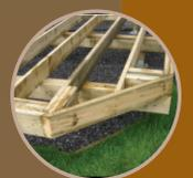
The anchor post connection is very strong. But it is useless if the anchor to deck connection is weak. The lag bolts or screws should penetrate deeply into solid wood and a solidly framed deck. For concrete or other hard surfaces, use proper fasteners.
