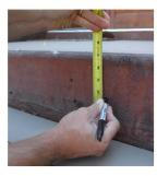
Determine where the fixture is to be installed and make a reference mark for drilling the 3" round hole. Tip: Measure from top of stair tread to bottom and divide this # in half and make a mark. Next, measure from left to right across stair tread and divide this # in half and mark. Center is where the two marks intersect.
