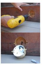
Drill a 3/8" hole all the way through the deck in the center of the 3" hole. Next, run the fixture wire through the 3/8" hole to underside of deck where wire connections will be made.
