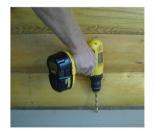
Drill a 3/8" hole through the deck surface and feed main line through to the under side of deck. Next, run the main wire to your first fixture. Secure the main wire using staples or cable tacks. Tip: For faster installation pre-wire the main run before decking is installed!
