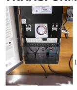
Using installation instructions provided with transformer, mount transformer to house and install main power feed line. This line should be a UV resistant, UL approved 12-2 low voltage line. Be sure main line is long enough to reach the first lighting fixture.
