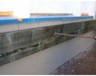
Remove ledger, center Deck2Wall Spacers™ over bolt holes and attach with corrosion-resistant screws or nails to the building side of the ledger.
